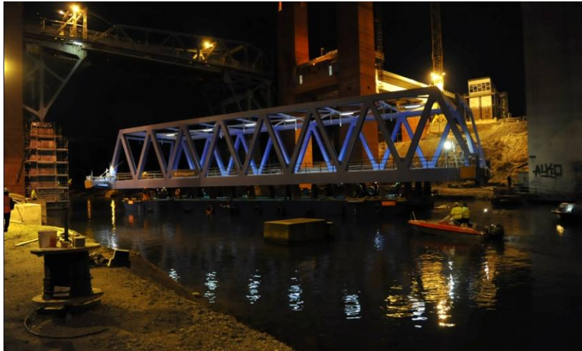
Barge with bridge transported in-between the pylons
