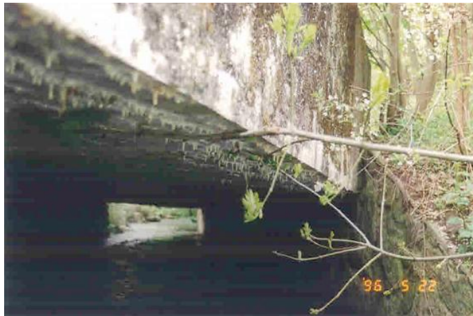
Underside af overbygning 1996
