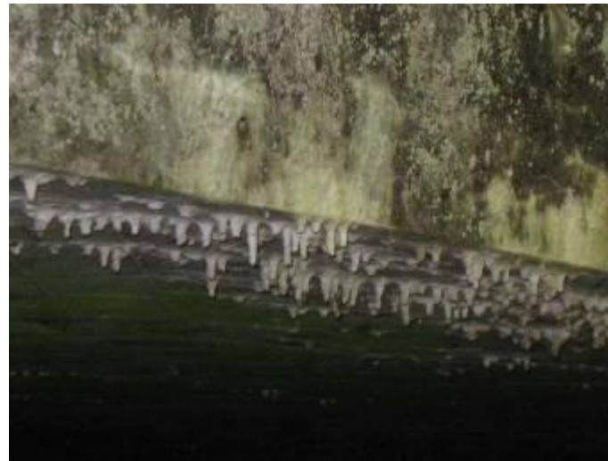
Underside af overbygning 2009
