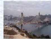
Ting Kau Bridge
