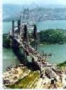
Kap Shui Mun Bridge
