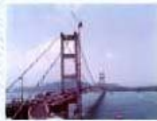
Tsing Ma Bridge
